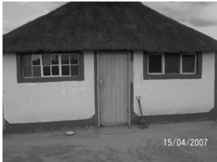
Fig 4. Roof supported by the walls
