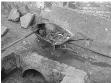
Figure 1: Exit from homes
