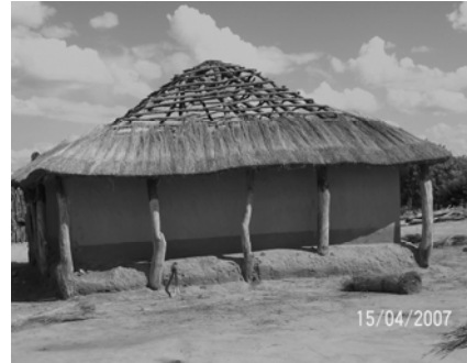
Fig 5. Cross beam technique of supports
