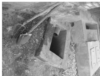
Figure 4: Exit from kitchen
